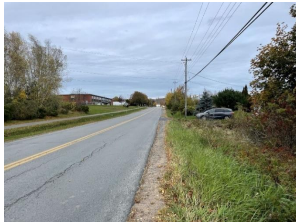
Figure 10: Southern access to J Jordan Road facing north
