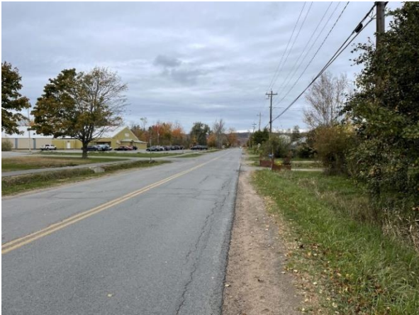
Figure 8: Northern access to J Jordan Road facing north
