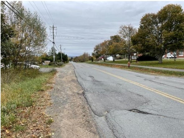
Figure 7: Northern access to J Jordan Road facing south
